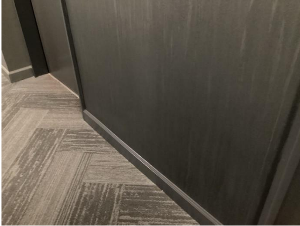
Recently installed wall coverings
