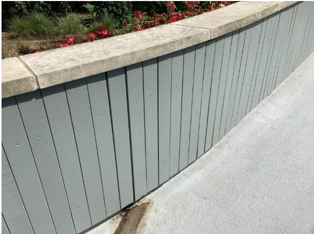
Wood siding at planter
