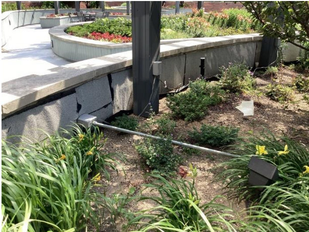
Membrane at perimeter at 2nd floor planter
