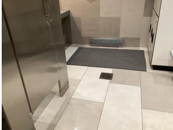
2nd floor rest room
