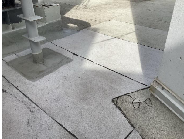
Tower roof system at repairs
