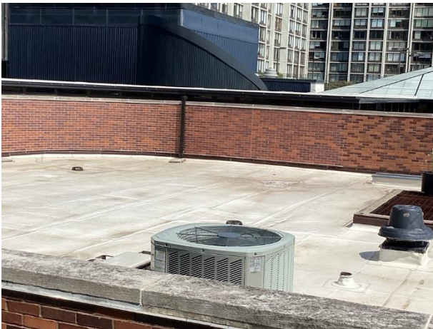
East or center roof at 2nd floor
