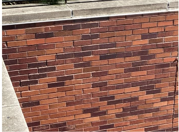
Masonry crack
