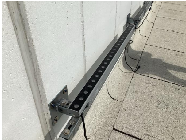
Light fixture mock up
