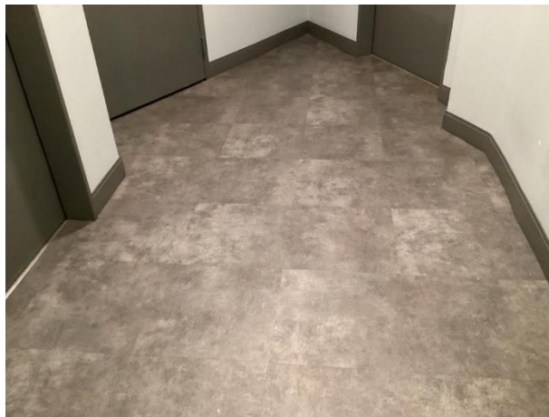
Service area flooring
