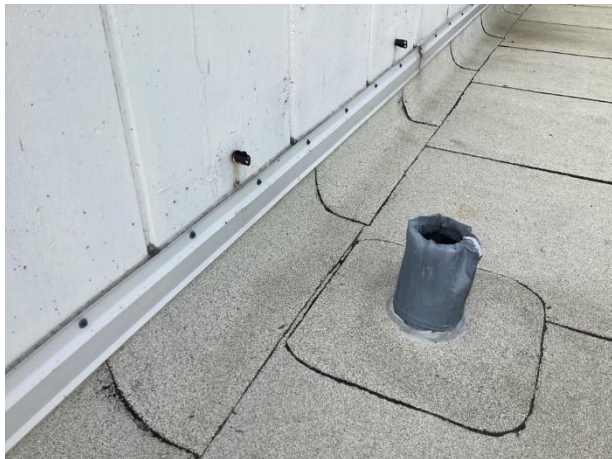
Penthouse roof at perimeter
