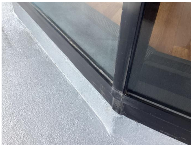
2nd floor common window system
