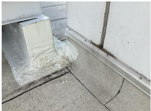
Tower roof system at perimeter
