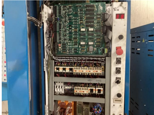
Traction elevator controls for high rise
