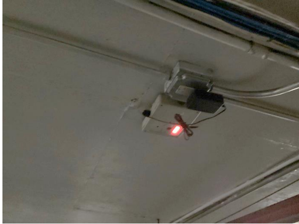
Carbon monoxide detector
