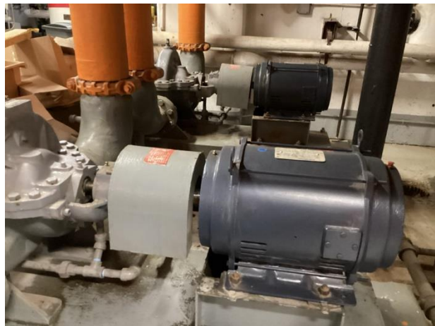
Commercial heat pumps
