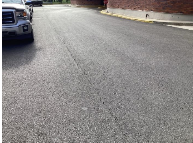
North perimeter pavement
