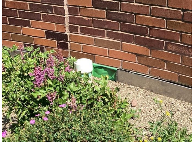
Flashing repairs at 2nd floor planter
