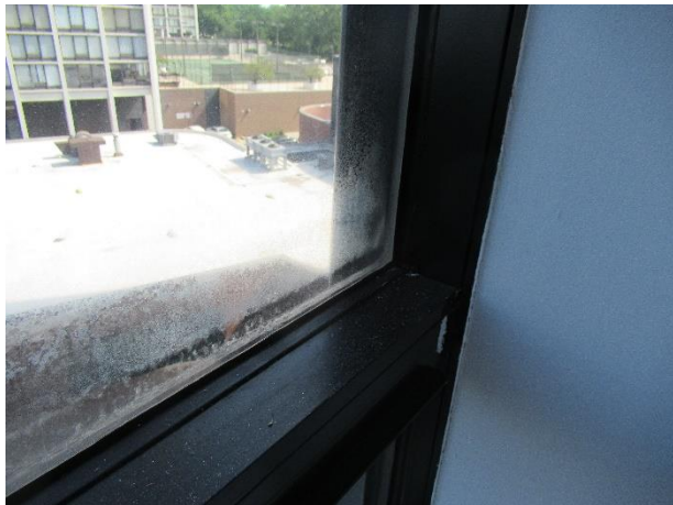
Curtain wall at interior seal
