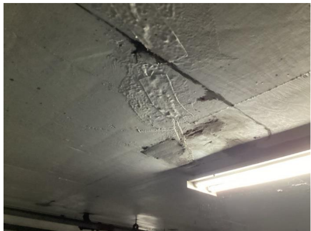
Typical repairs beneath plaza
