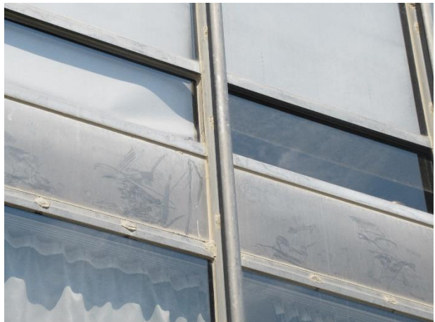
Spandrel panel conditions
