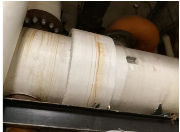
Main building heat exchanger
