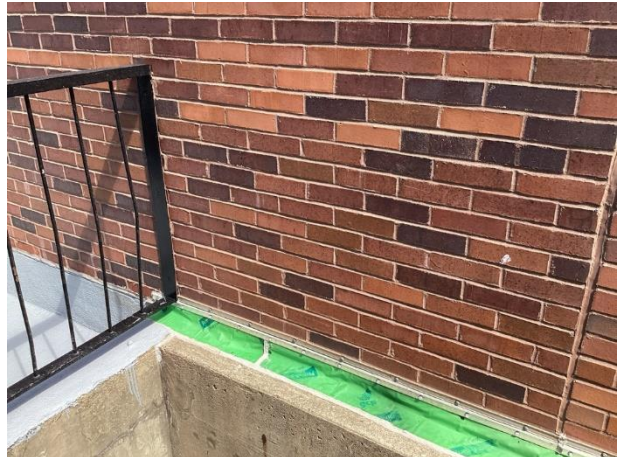
Recent masonry repairs and flashing installation
