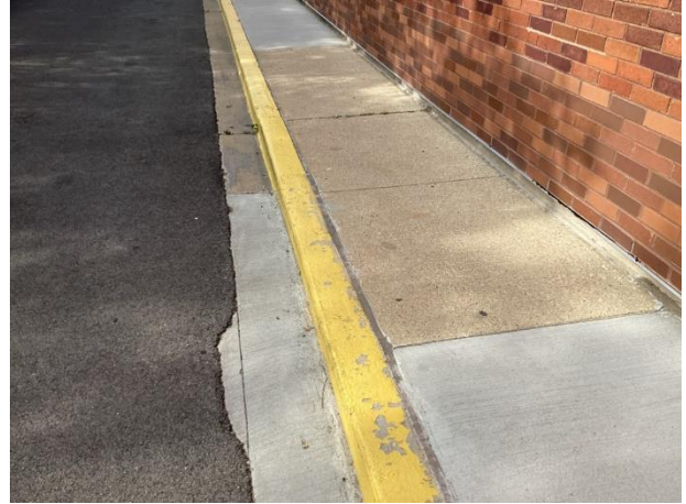
Varied sidewalk replacements
