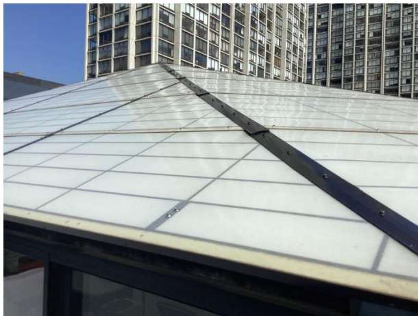
Pool enclosure roof
