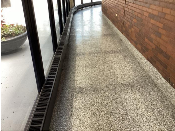
Coating at floor at walkway
