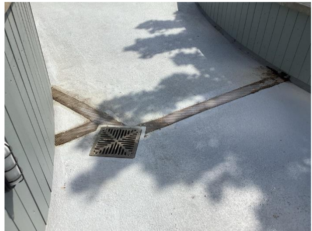
Waterproof coating at drains at 2nd floor roof
