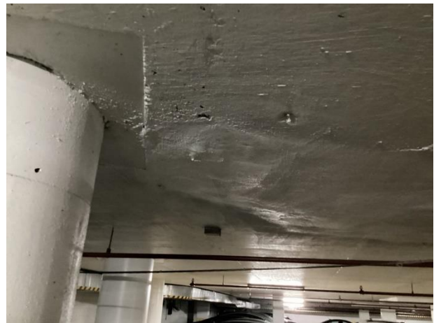
Repairs beneath elevated floor
