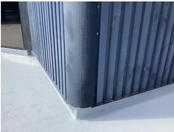
Metal siding at base
