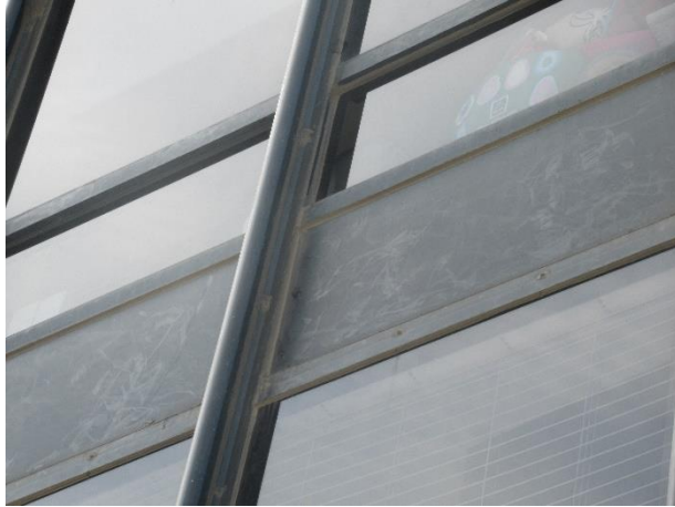
Spandrel panel conditions
