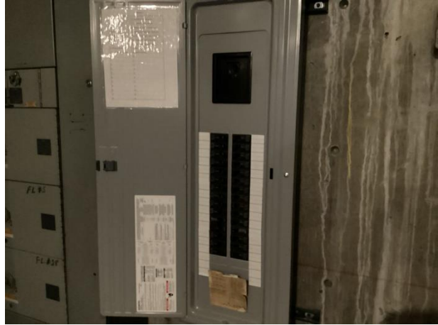
Replaced circuit protection panel for garage
