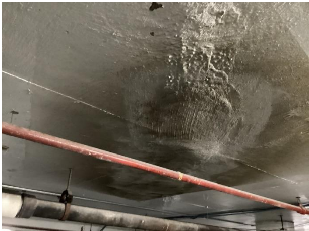
Repairs beneath plaza
