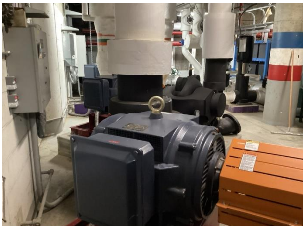
Dual temperature pumps
