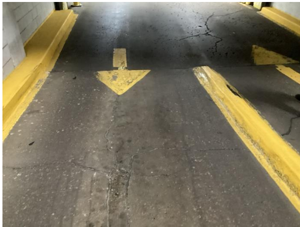
Concrete cracks
