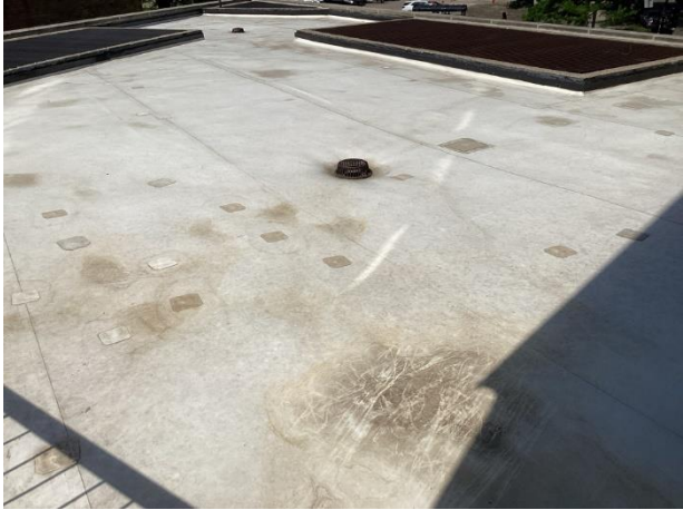
Southwest 2nd floor roof system at repairs
