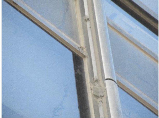
Glass/metal and metal/metal sealants
