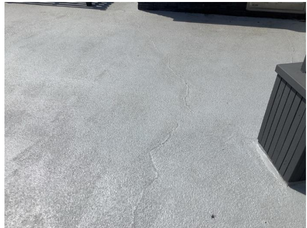
Concrete repairs beneath traffic coating at 2nd floor roof
