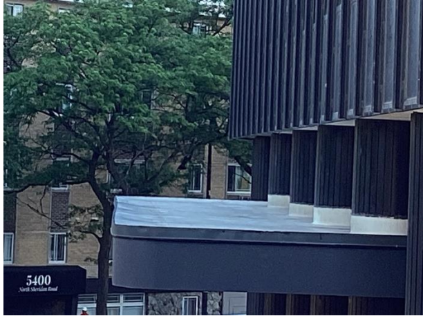
Lobby canopy roof
