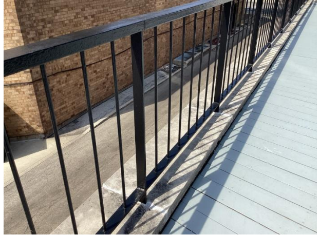
Steel railing at south perimeter of 2nd floor
