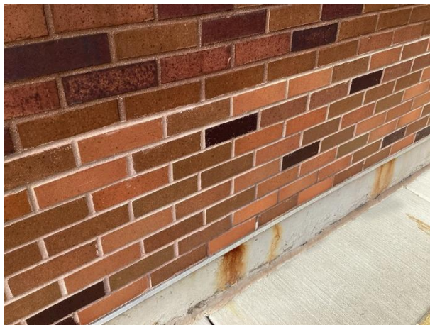
Replaced masonry and flashing installation
