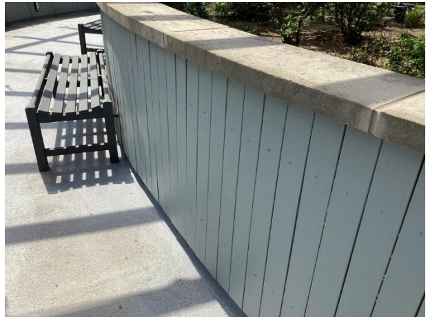
Siding at planter at 2nd floor
