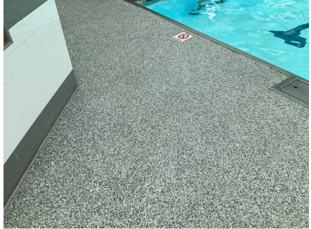
Pool deck coating
