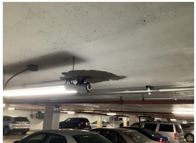
Typical repairs beneath elevated floor
