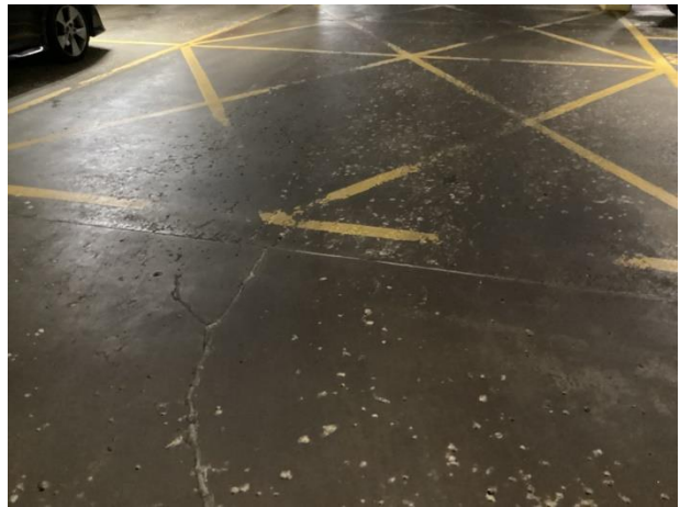
Concrete spall
