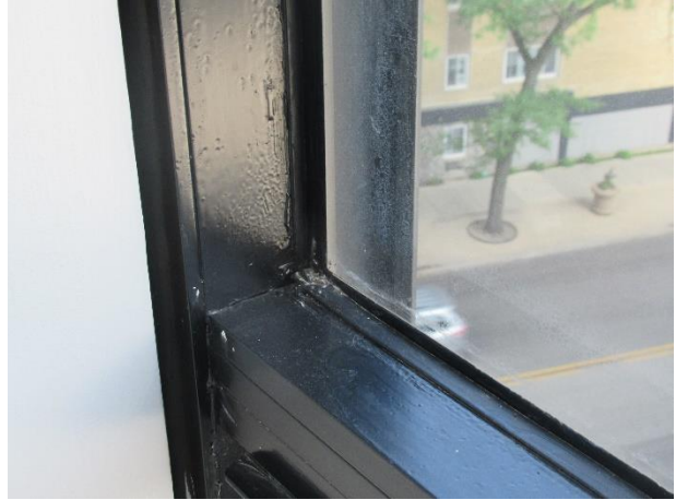
Curtain wall at interior seal
