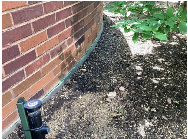
Perimeter flashing at 2nd floor planter
