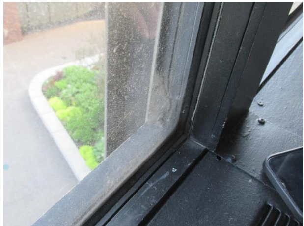
Curtain wall at interior seal
