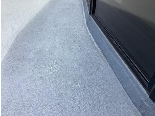
Waterproof coating at perimeter at 2nd floor roof
