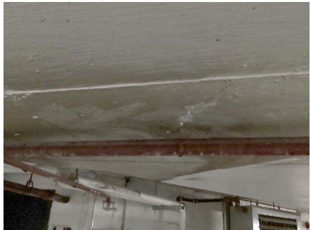
Repairs beneath plaza
