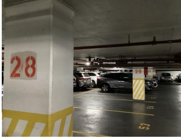
Garage paint finishes overview
