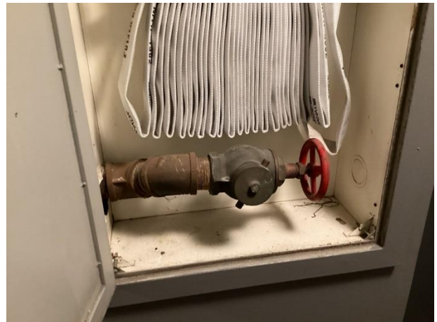
Valve for standpipe
