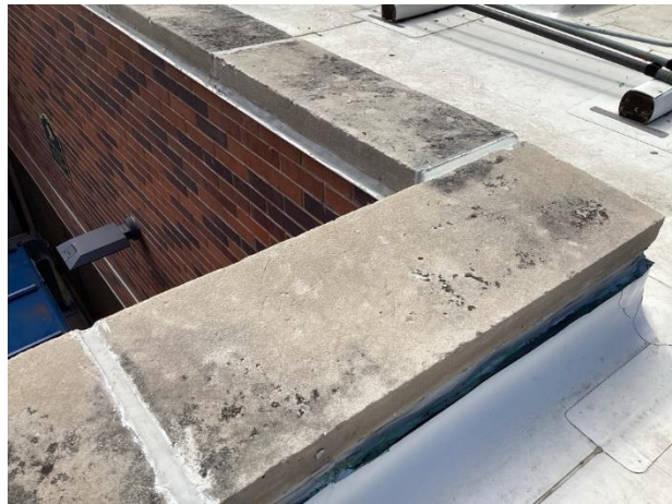
Flashing at wall caps
