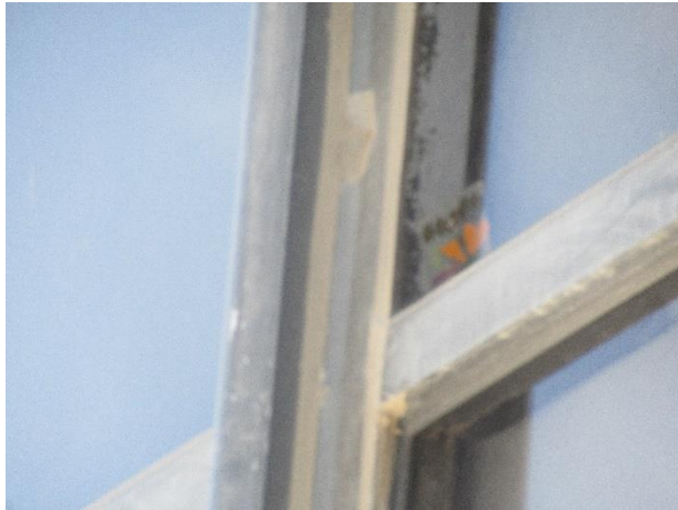
Glass/metal and metal/metal sealants
