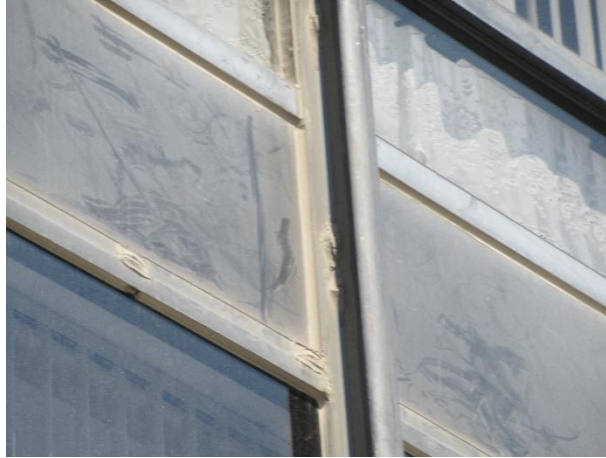
Spandrel panel conditions
