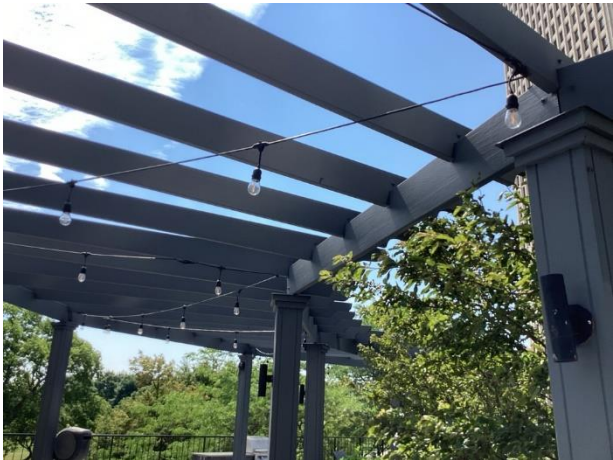
Pergola at 2nd floor
