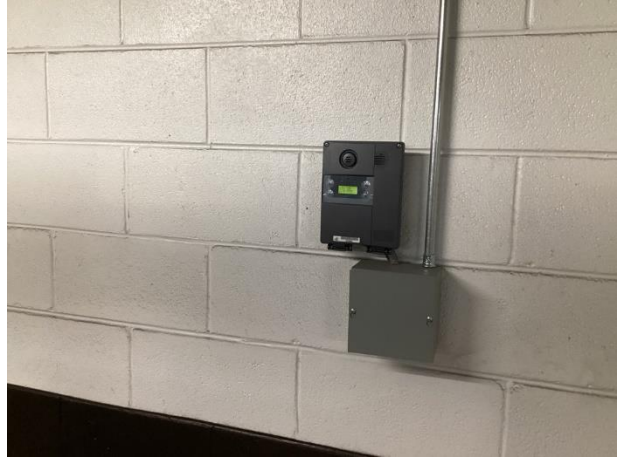
Carbon monoxide detector
