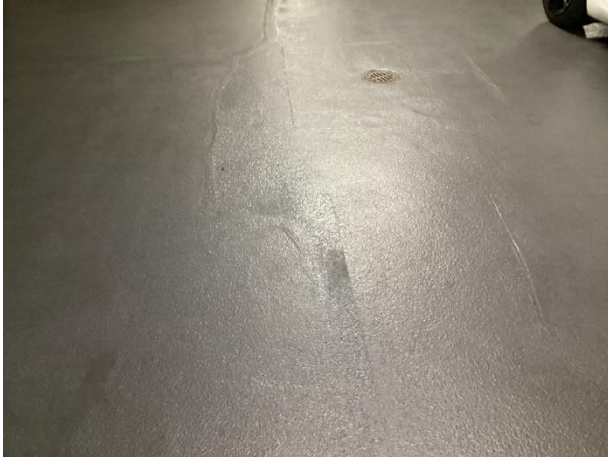
Repairs beneath traffic coating
