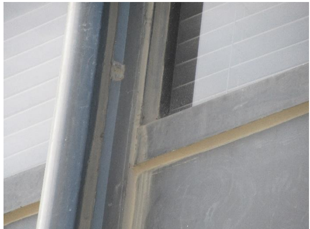
Glass/metal and metal/metal sealants
