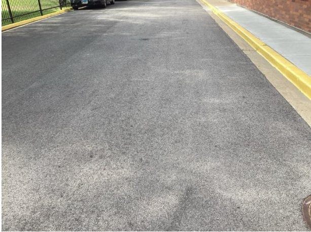
East perimeter pavement
