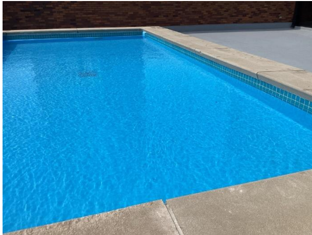
Outdoor pool plaster finish
