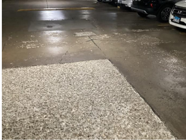
Concrete spall
