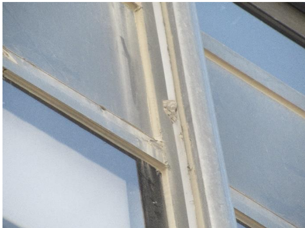
Glass/metal and metal/metal sealants
