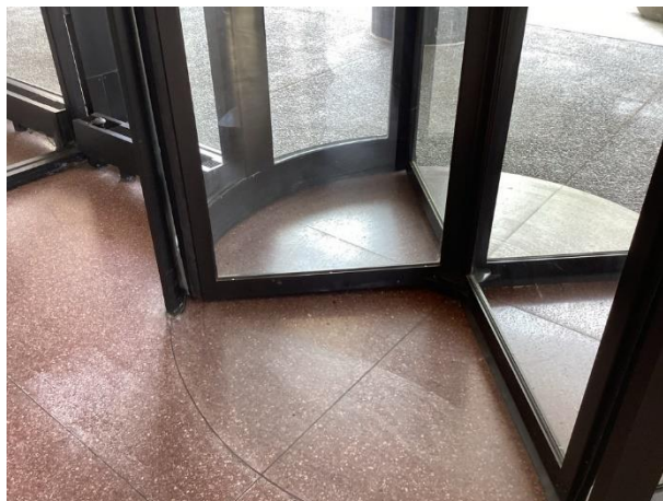
Recently replaced revolving door
